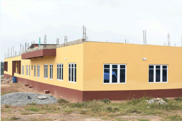
Completion of Phase-1 of the Faculty of Medical Rehabilitation Building
